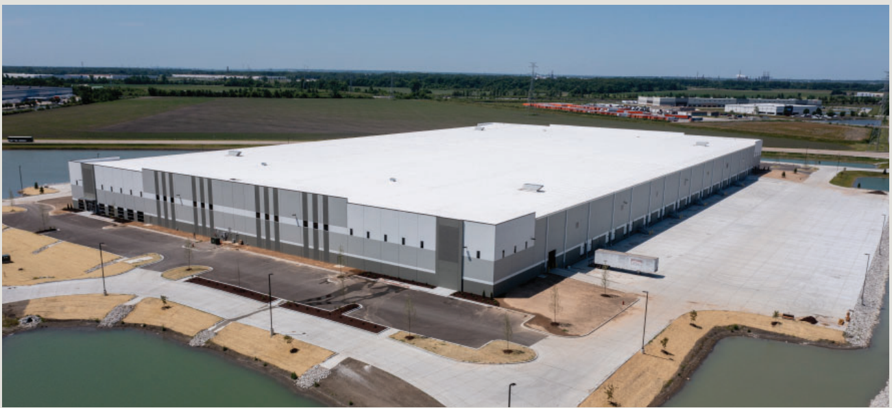
Panattoni leased 455,900 SF, one of its two buildings to WorldWide Technologies, located in Gateway Commerce Center.
