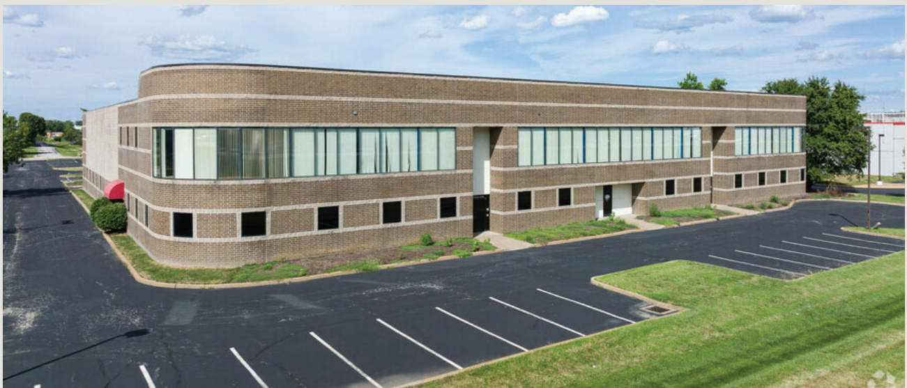
Jeff Hawley and Brandon Duncan represented Window World in the purchase of 3600 Rider Trail, a 49,950 SF Office Warehouse Building.
