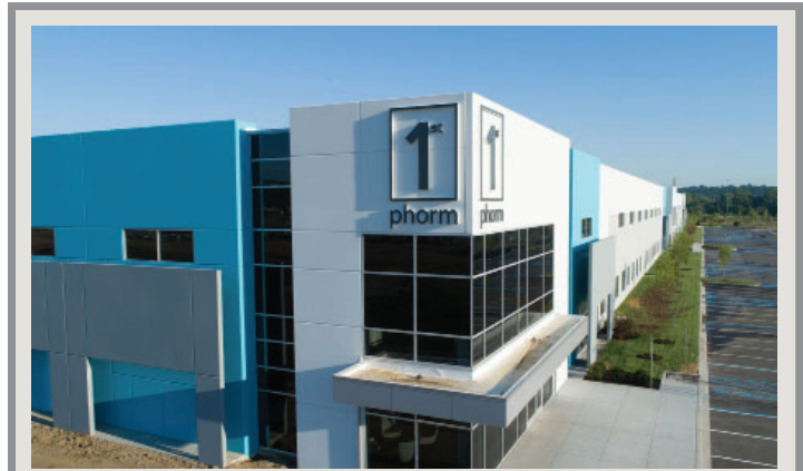
U.S. Capital Development delivered the 182,000 square foot 1st Phorm building at Fenton Logistics Park.
